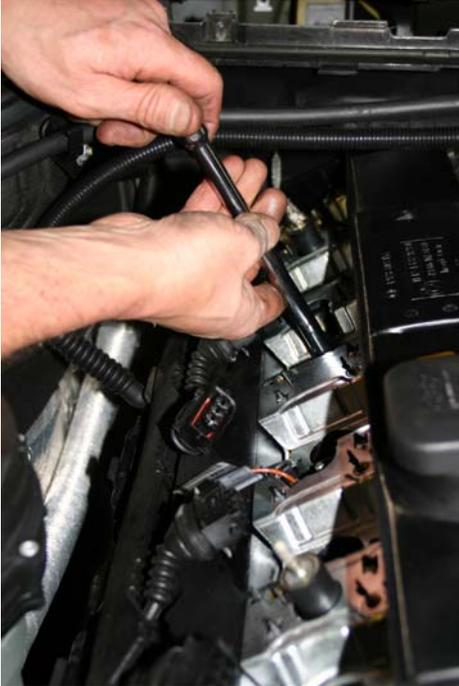
Replacing spark plugs in an M54 engine.
